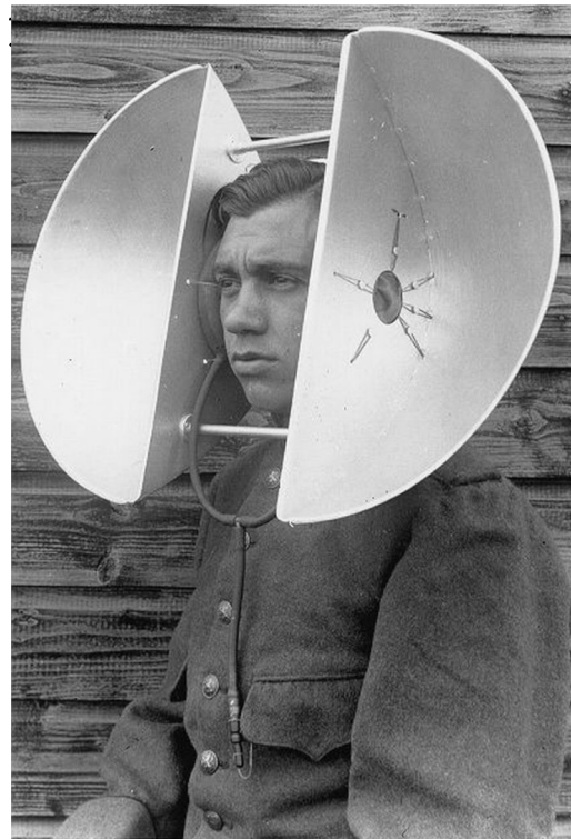
Fig. 3: Topophone (left), Patent No. US590062, WWII Military Bomber Detector.
